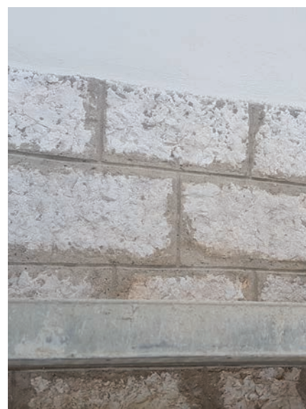
hydrogommage (nettoyage) des joints existants
