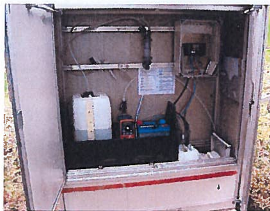
Chloration provisoire
